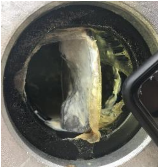
Contaminated pipe (binder) before procedure
